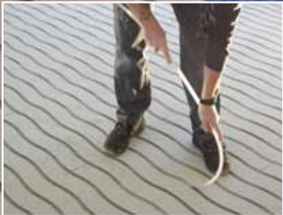
The plastic pipe is placed into the grooves.
