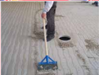
The protruding body filler will be removed from the supporting panel.
