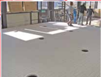
After the operational heating the MERO Combi T Thermo is ready for the application of the floor covering.
