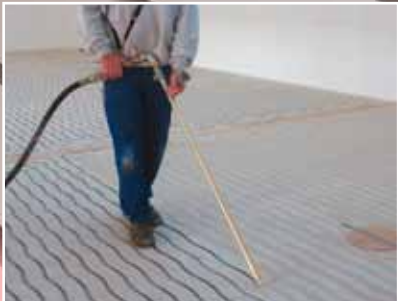
Prior to the grouting of the body filler, all pipes are tested for leaks.
