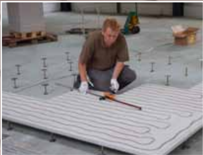
The MERO dry hollow floor with pre-fabricated grooves for the heating pipes is installed according to the layout drawing.
