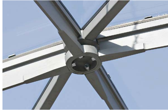
Figure 28. End-Face Connector MERO-4*
