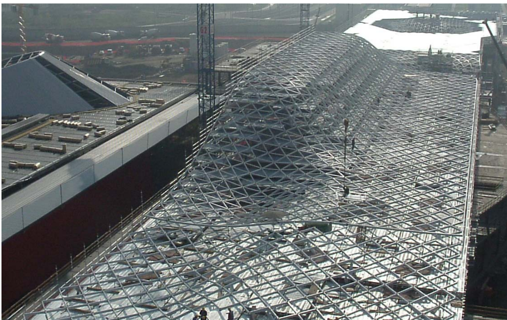
Figure 30. New Fair Milan, Roof over the Central Axis during Construction
